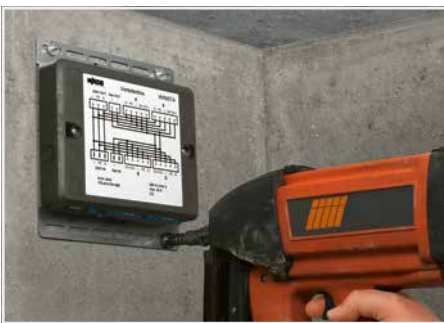
Securing the mounting plate with WINSTA® Box to the wall (e.g., via stud gun).
