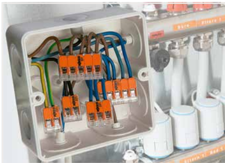
Wiring Fine-Stranded Conductors in Junction Boxes
