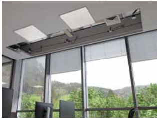
Installation of Shading Systems
