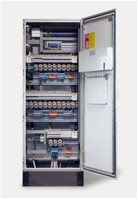
Works photo, WAGO
