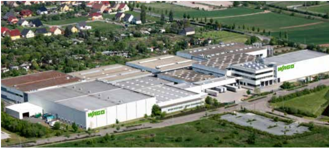
WAGO Sondershausen, Germany
