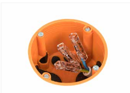
Extending short wires.
