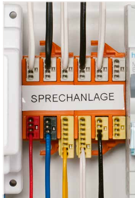
Example of a residential intercom application
