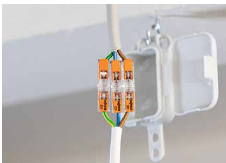
Lighting connection in suspended ceilings
