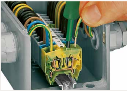
CAGE CLAMP® connection Inserting a conductor. With ferruled conductors, it is necessary to use a terminal block one size smaller than the conductor's nominal cross-section.
