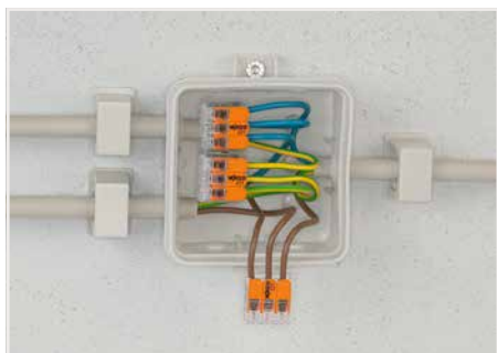
Wiring fine-stranded conductors in a junction box.
