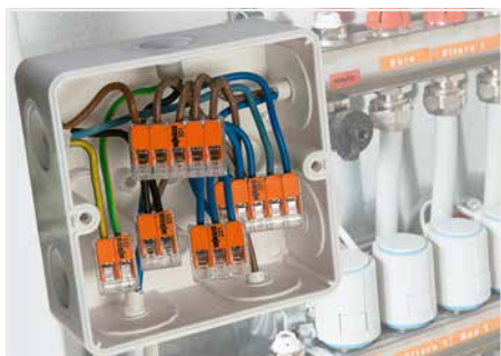
Wiring fine-stranded conductors in a junction box.
