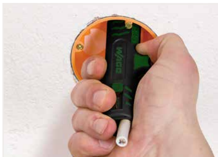
Stripping a cable sheath.
