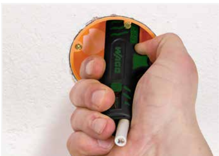
Stripping a cable sheath.
